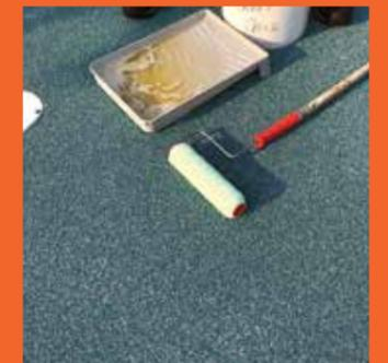
Sealing the surface with aliphatic top coat.
